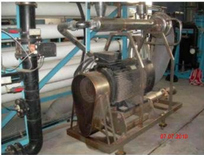
Reverse Osmosis Pressurizing System, Sea Water Desalination Plant, Deir Al Balah governorate
