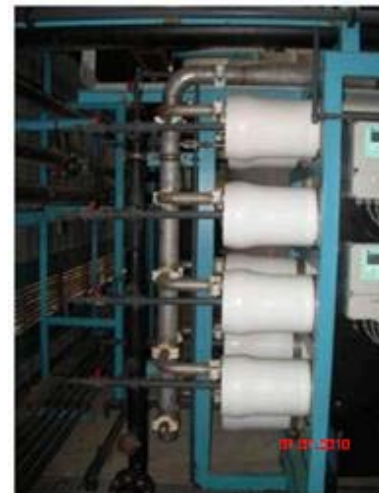
Reverse Osmosis System, Sea Water Desalination Plant, Deir Al Balah governorate
