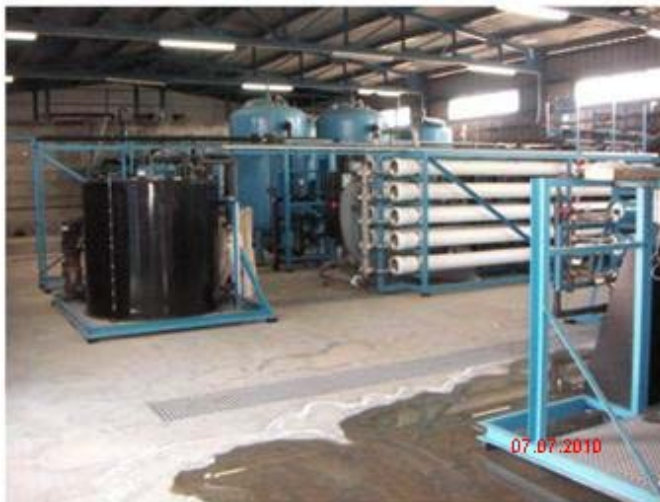
Reverse Osmosis System, Sea Water Desalination Plant, Deir Al Balah governorate
