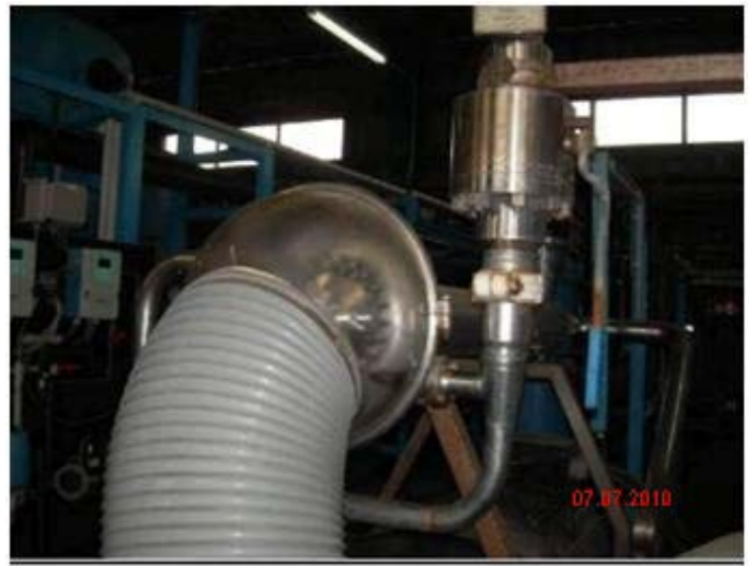
Reverse Osmosis Pressurizing System, Sea Water Desalination Plant, Deir Al Balah governorate
